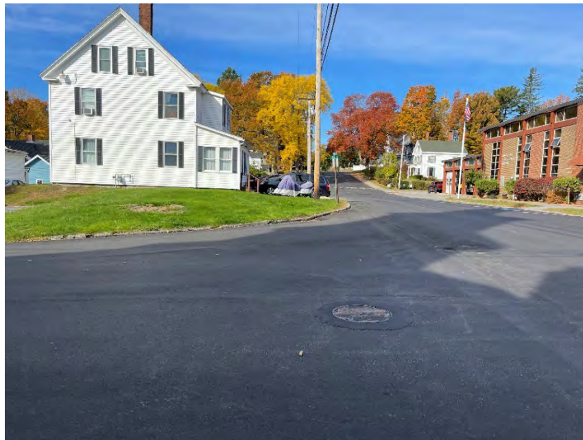
Looking west from Elm Street along Franklin Street
