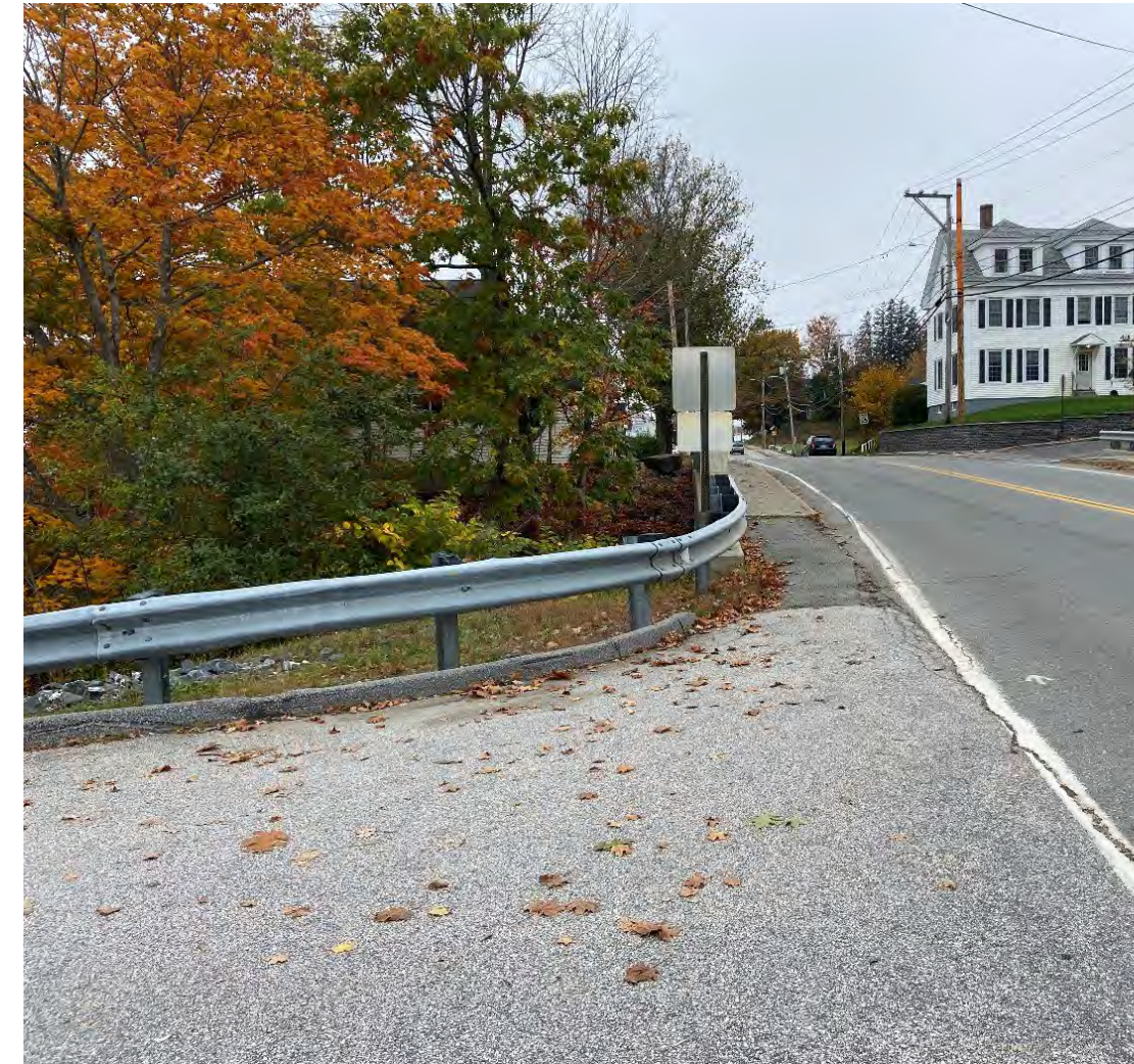
Looking west along Main Street from Veterans Park
