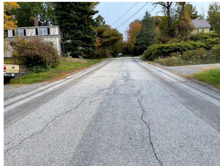
Looking up 2nd Street from Main Street
