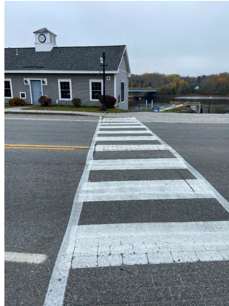
Crosswalk at Pine Street
